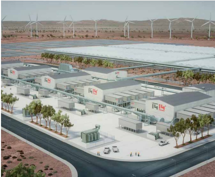
The Thermal Energy Storage System from 1414 Degrees uses electricity to heat silicon containers and then recover the energy stored to make electricity and heat.
