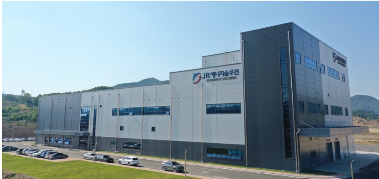
Figure 2 JR Energy Solution battery foundry in Eumseong, South Korea
